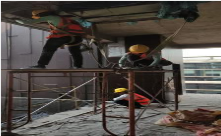
L-16-Safety installation on 04-03-23
