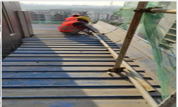
L-16-Safety installation on 06-03-23
