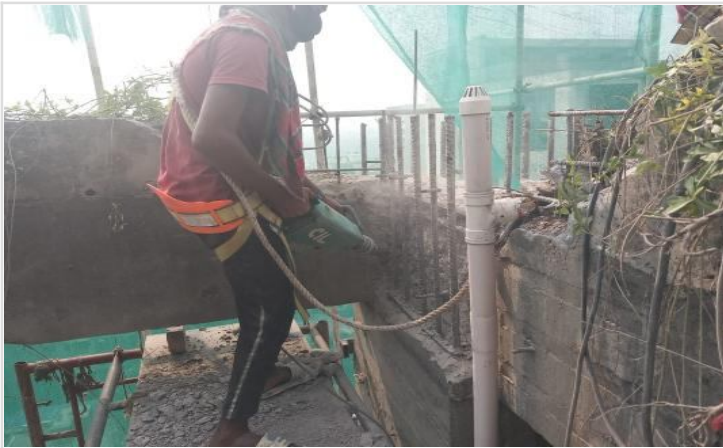
L-16-Old concrete removing on 22-03-23
