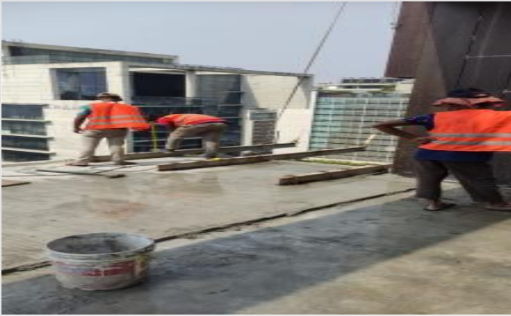
L-16-Safety Installation on 01-03-23
