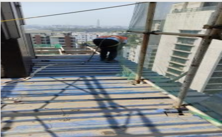
L-16-Safety installation on 06-03-23
