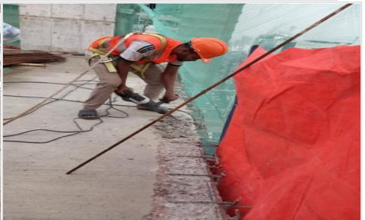
L-16-Dropwall old concrete dismantling on 29-03-23
