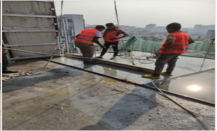
L-16-Safety Installation on 01-03-23
