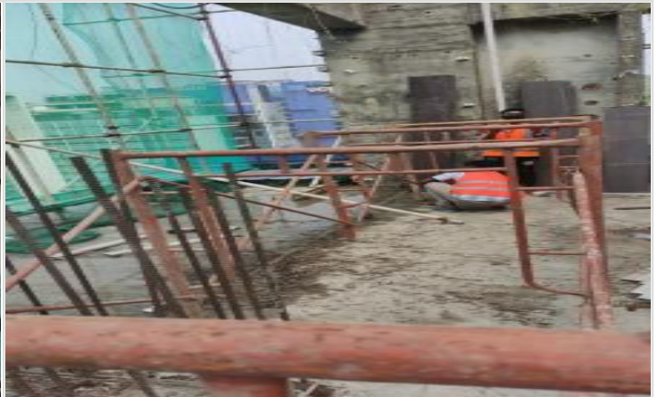
L-16-Safety installation on 18-03-23
