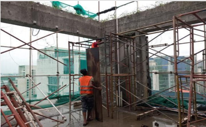
L-16 Scaffolding on 20-03-23
