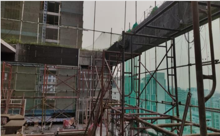
L-16-Safety installation on 18-03-23
