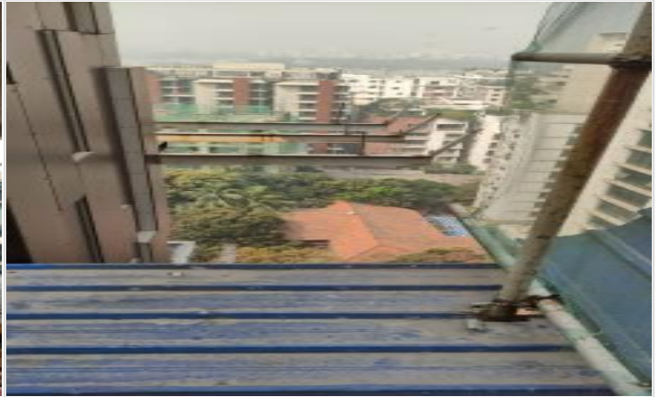
L-16-Safety installation on 04-03-23
