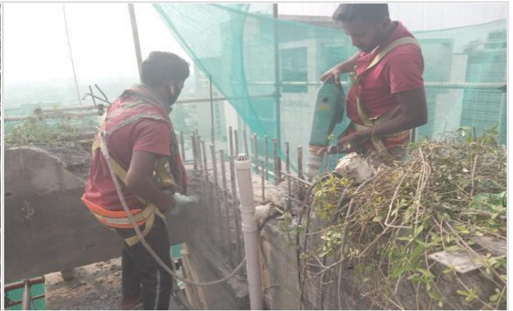
L-16-Old concrete removing on 22-03-23
